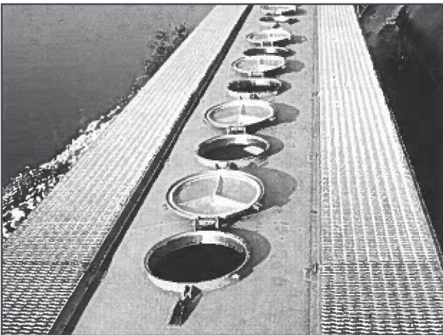
Wipe hatch rings, covers, and gaskets clean to assure proper sealing of covers.
